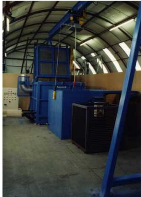
Aluminium heat treatment complex
